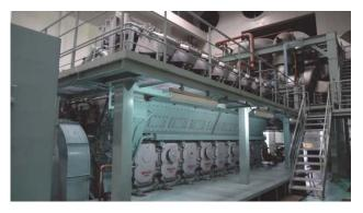
[Figure 1] Diesel-powered engine generator
