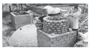
Figure 5: Construction of biodigesters in Cambodia through the National Biodigester Program (NBP, n. d.)
