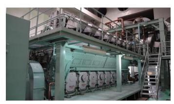
[Figure 1] Diesel-powered engine generator
